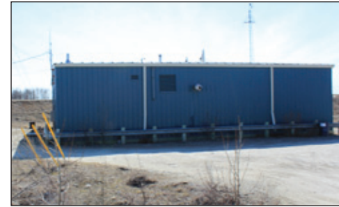
Fig. a262 - Municipal building
