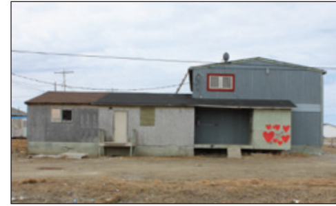
Fig. a117 - Previously the NAPS station, currently abandoned
