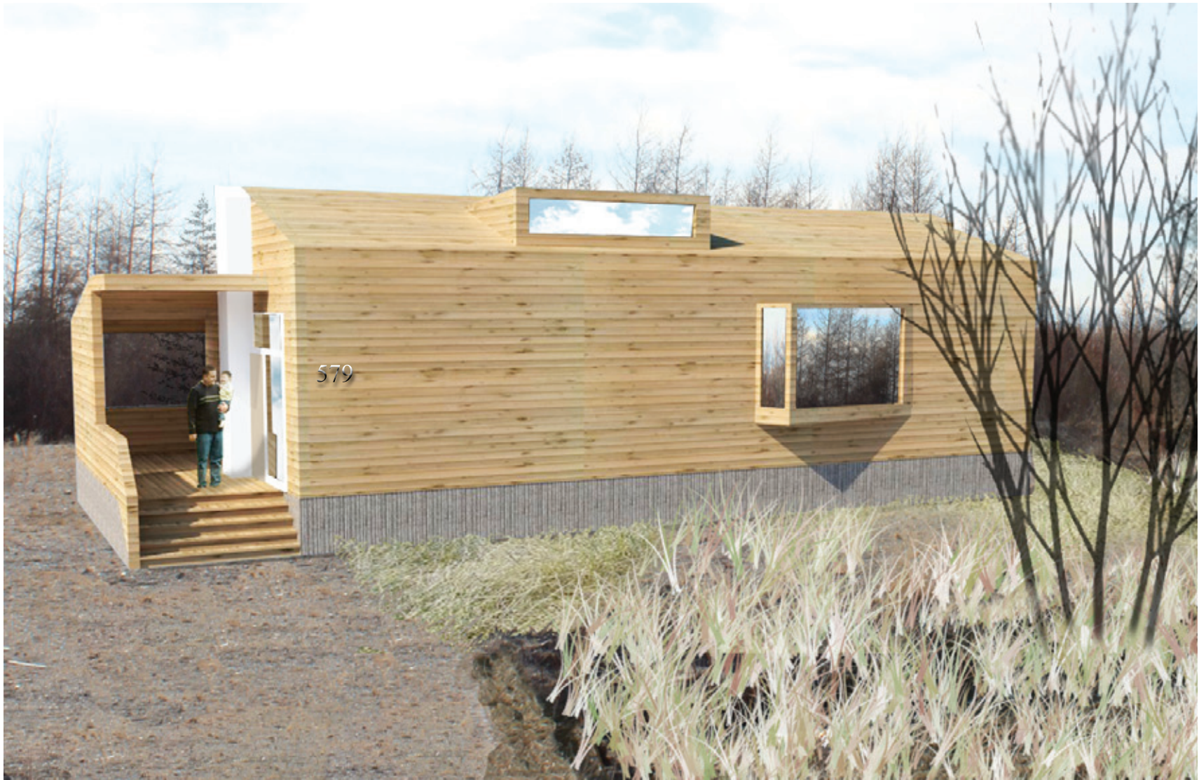
Fig. 39a - Treated pine is used extensively throughout both the interior and exterior of the house, creating an enveloping feeling with the simple beauty of wood. The vertical guidance sleeves are expressed on the exterior, while a generous porch allows items to be stored outside to float during a flood as well as for social gathering during the summer.
