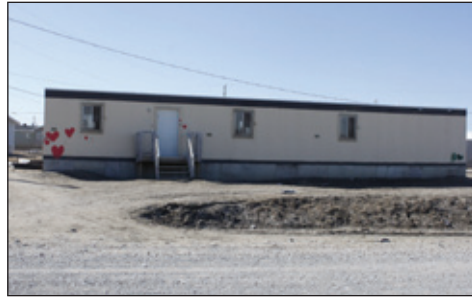
Fig. a29- Offices
