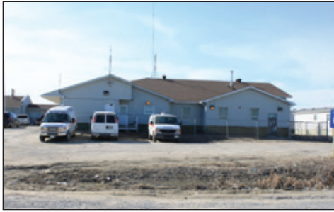
Fig. a205 - Nursing station buildings
