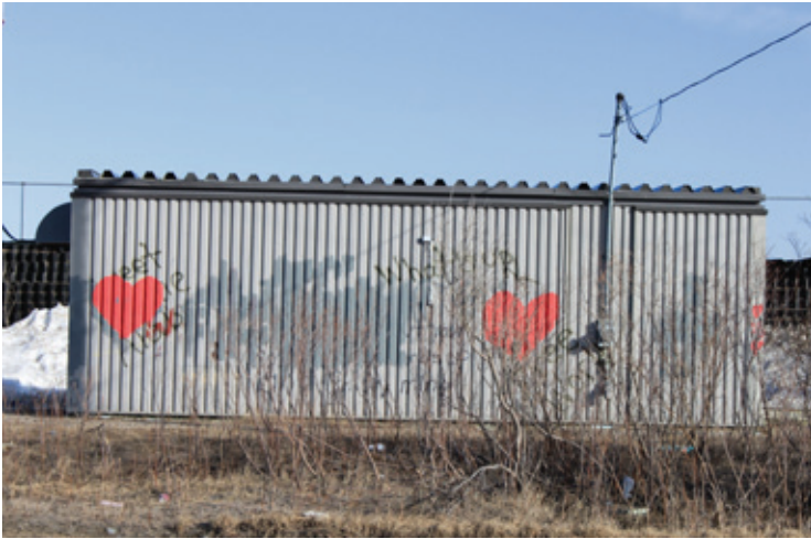
Fig. 21 - Water treatment facility located in the north east corner of the dike.
