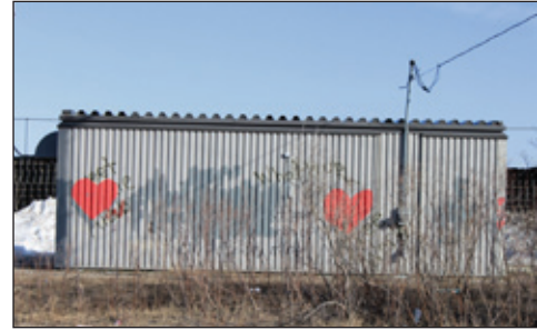
Fig. a239 - Water intake facility
