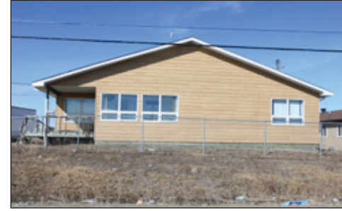
Fig. a203 - Nursing station building
