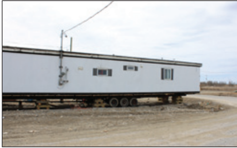
Fig. a87 - Trailer/Office
