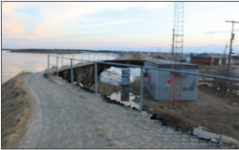
Fig. a242 - Water intake facility
