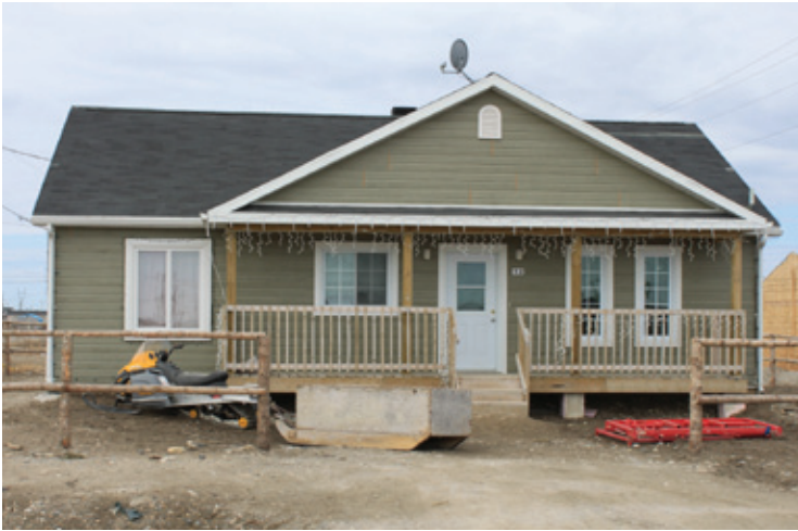
Fig. 14 - Newest housing development style where we stayed for the duration of our trip. This house represents the 'highest quality' of housing on many of the reserves in northern Ontario.
