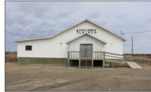
Fig. a94 - Community Church with accessible ramp
