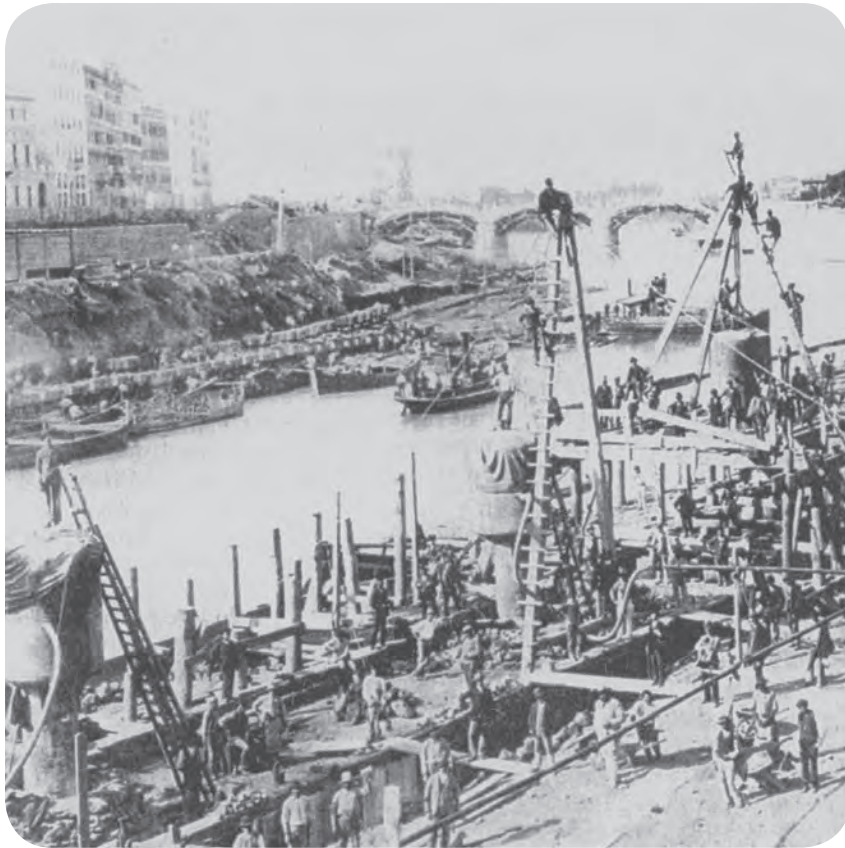
fig. 2.17 Construction of the Canevari's embankments, 1887.
