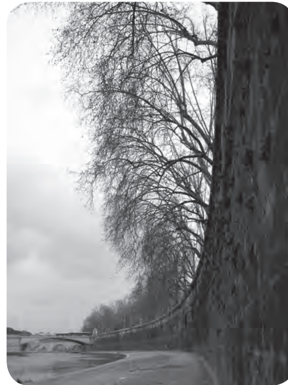
fig. 2.13 Canevari's embankment wall.
