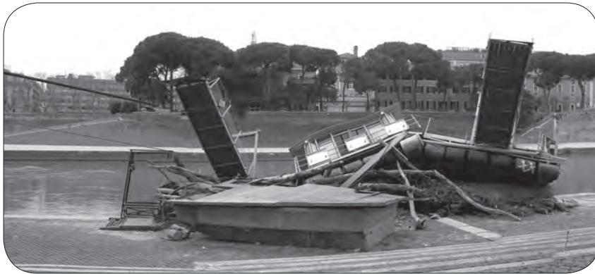
fig. 1.91 The aftermath of the December 2008 inundation, three months later.
