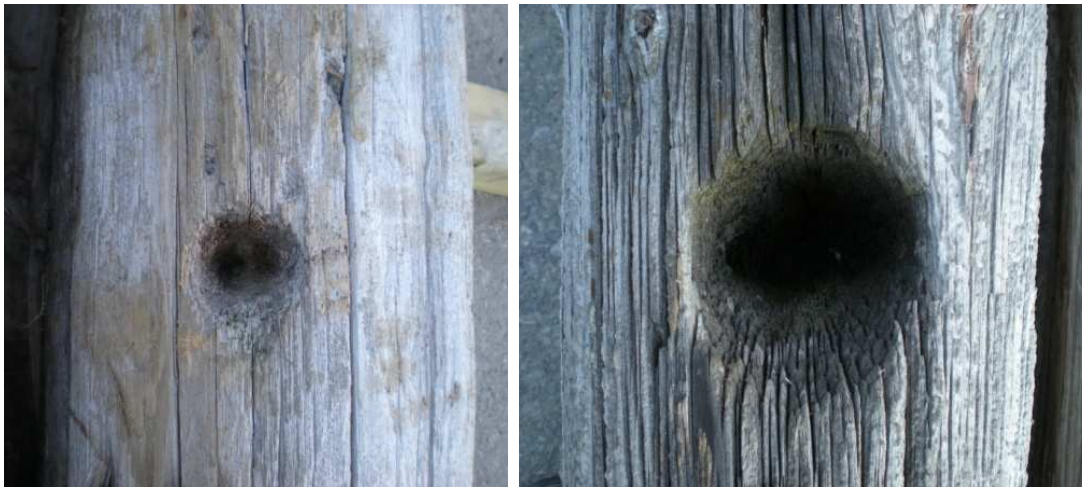
Figure 10. - In-service exploratory damage (left) and feeding damage (right).
