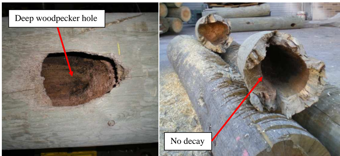
Figure 75. - In-service specimen with nesting level woodpecker damage and no decay (RP-3-1).
