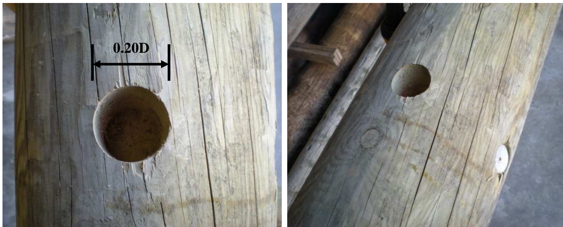
Figure 17. - New pole specimen idealized exploratory damage.
