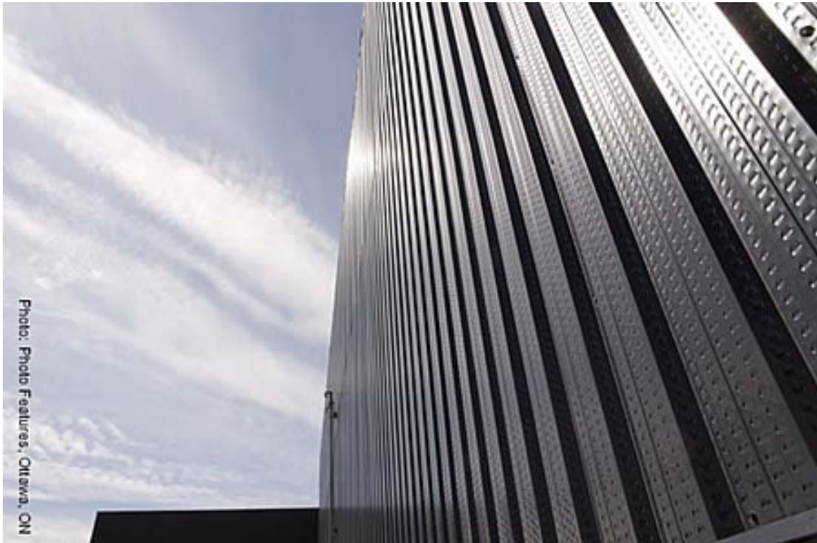
Figure 1.6: An Unglazed Transpired Solar Collector (NRCan 2009).
