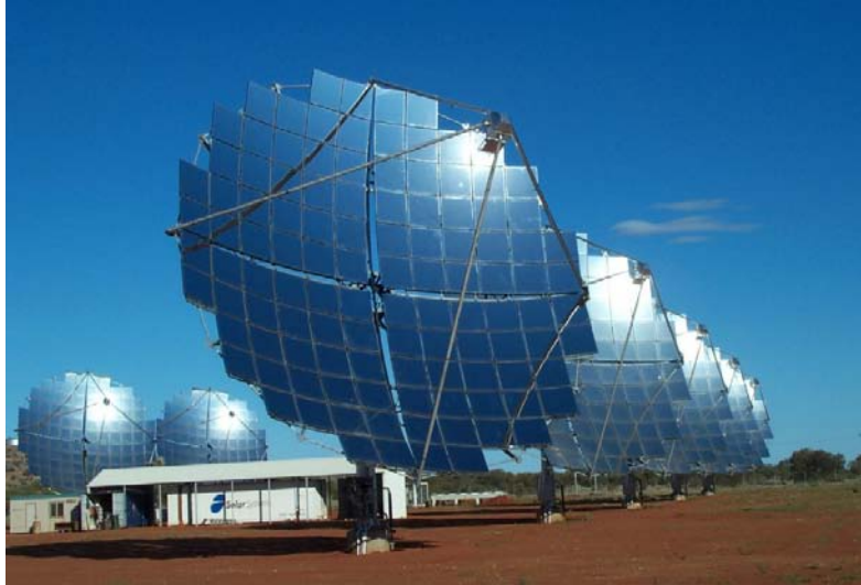
FIGURE A.2 - PARABOLIC DISH CPV COLLECTOR (DESERTEC-UK 2009)
