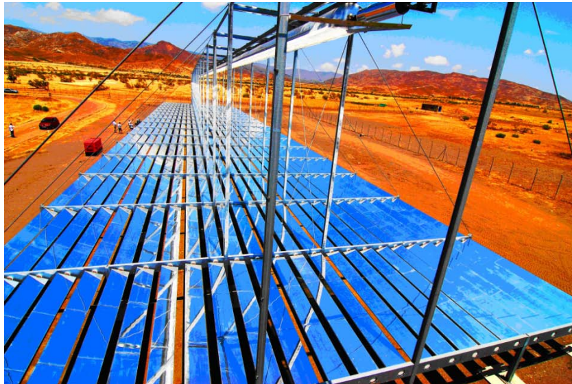
FIGURE A.3 - LINEAR FRESNEL COLLECTOR (DESERTEC-UK 2009)
