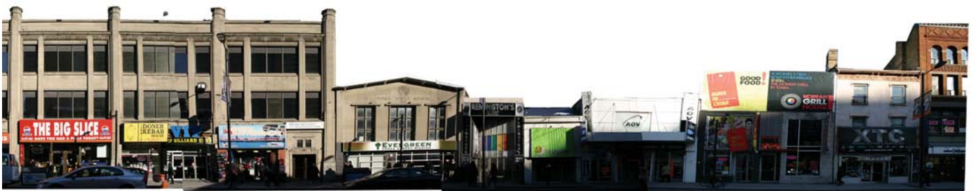
Fig. 1.16 West facing elevation of Yonge Street just south of Gerrard Street.
