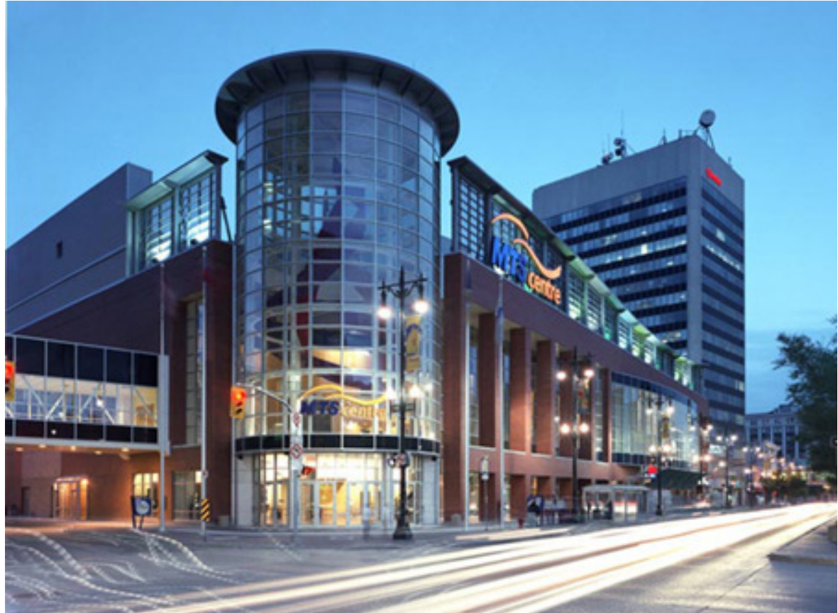
Figure 2.6.5: MTS Centre as built
