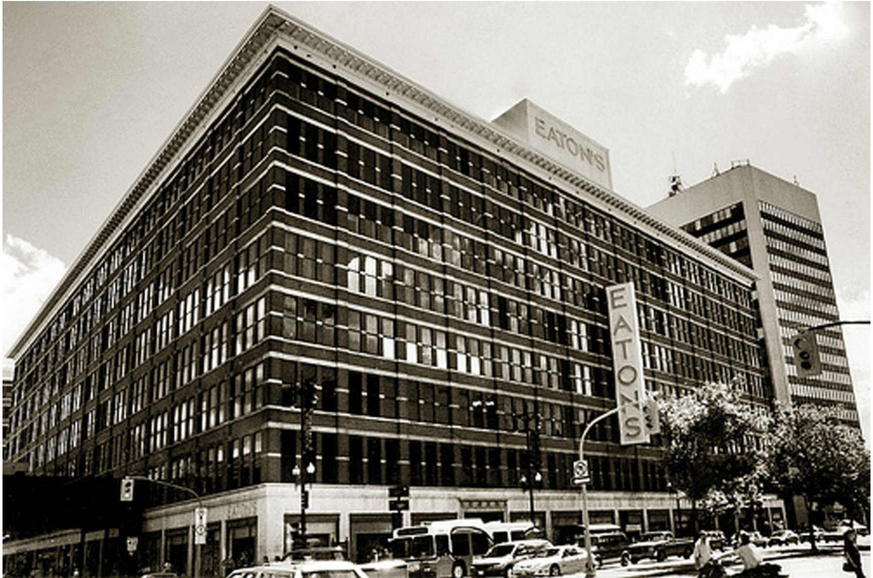
Figure 2.6.3: Old Eaton Building
