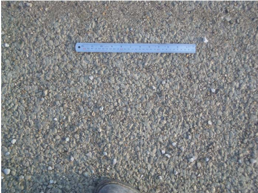
Appendix A-15 Permeability Rating: Fair.
