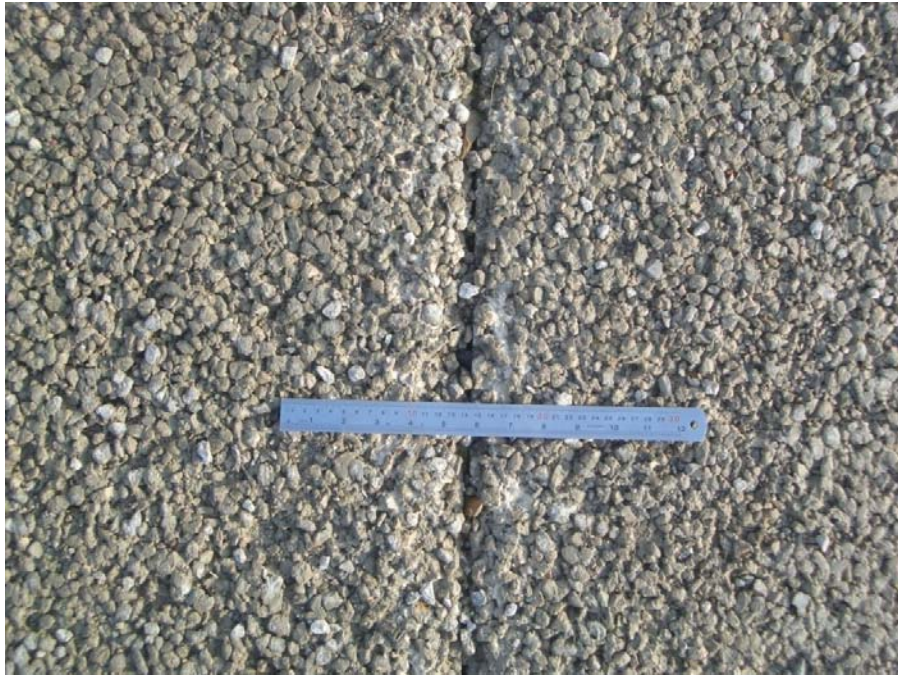
Appendix A-5 Surface Distress Rating: Good (Close View).
