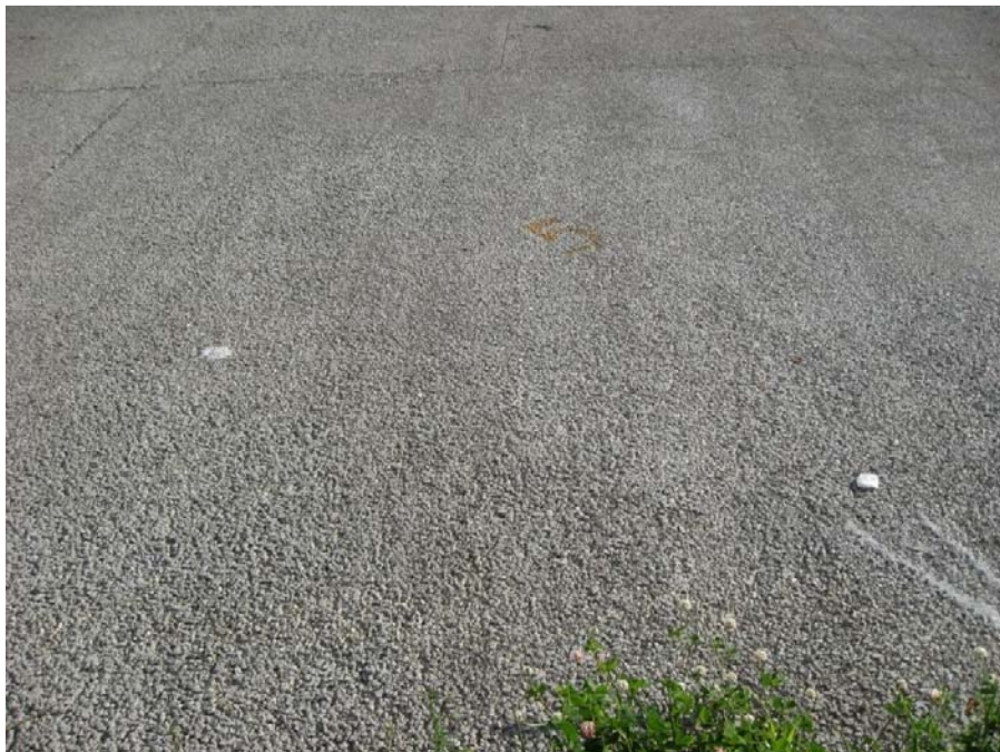
Appendix A-6 Surface Distress Rating: Good (Overall View).
