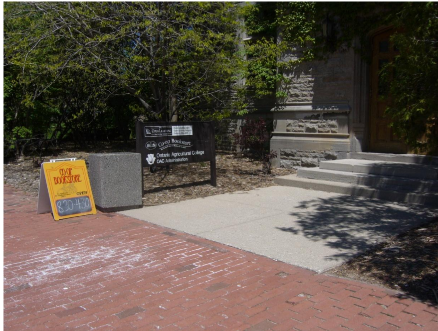
Image 1: Lack of Ramp to Access Campus Co-op Book Store
