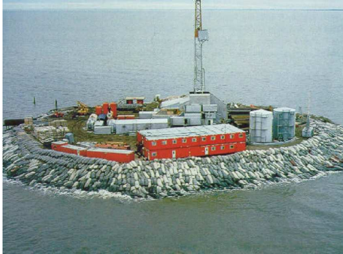
Figure 5.3: Picture of an artificial island with a sandbag protected shoreline (from Timco and Johnston (2002)).
