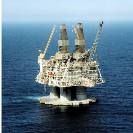
Figure 5.4: Aerial photograph of Hibernia GBS off the Grand Banks of Newfoundland, a bottom mounted structure (from Hibernia (2009)).
