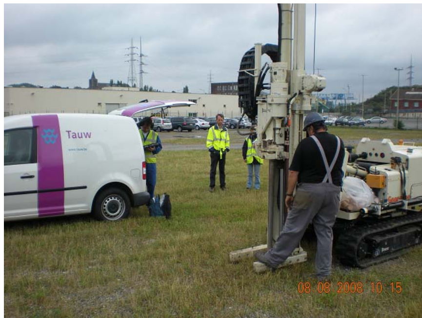
Figure 7-1: Field personnel coring a hole for the deployment of TWA-PDMS samplers and GORE™ Modules
