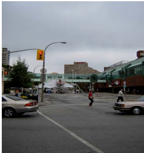
Figure 57, Street Light, Kitchener
