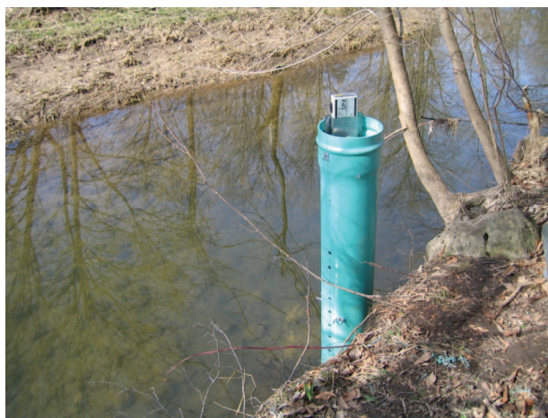
Figure A.3: Float Installation - West Sub-Basin (14-Apr-2005)
