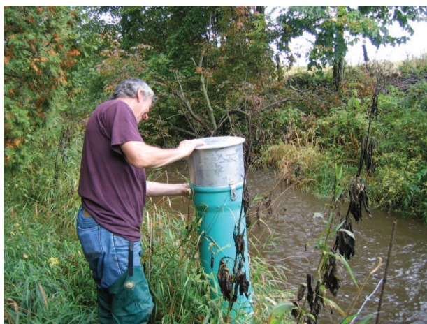
Figure A.2: Float Installation - East Sub-Basin (26-Sep-2005)
