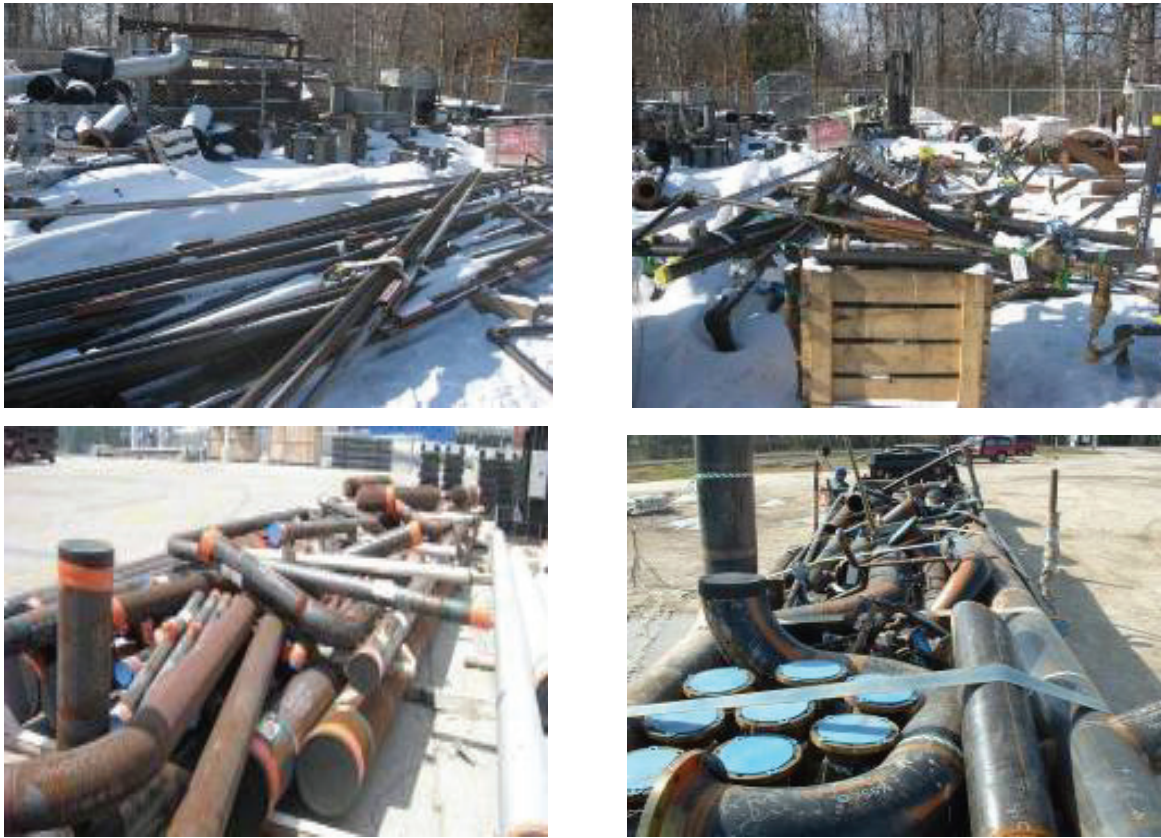
Figure 4.6: Examples of materials storage at Portland Energy Centre site
