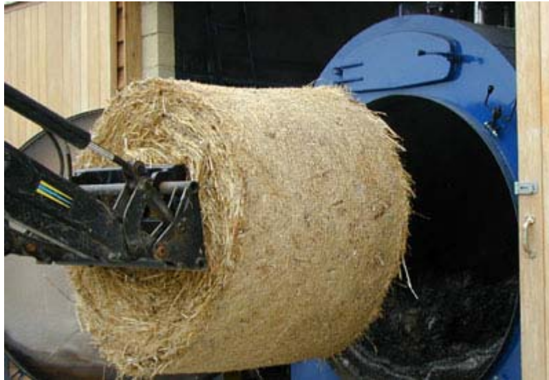
Figure 2.2: Heavy Equipment Stoking (Northmoor Trust 2008)
