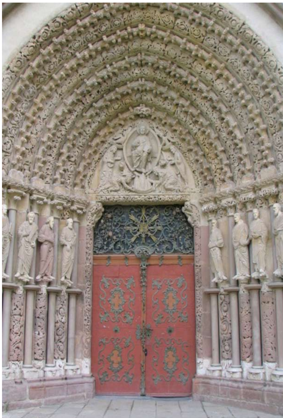
3.16 Former Cistercian nunnery, Porta Coeli in the Svatka Valley outside of Brno, Czech Republic
