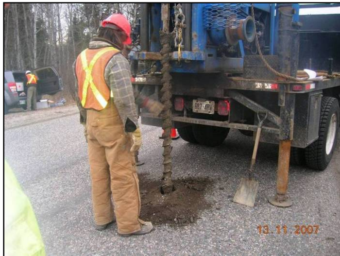
Figure 4.2: Coring for Thermistor Installation.
