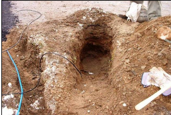
Figure 4.5: Installation of CS-616, the probe is inserted into the subgrade, Hwy 651
