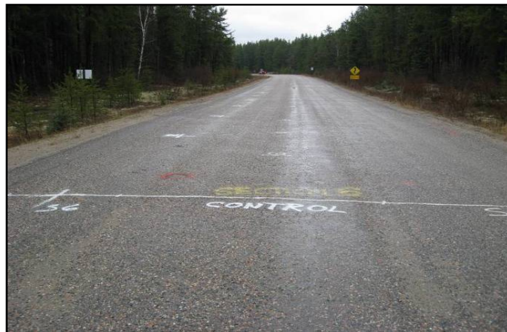
Figure 3.17: Highway 651, Section 6-Control Section
