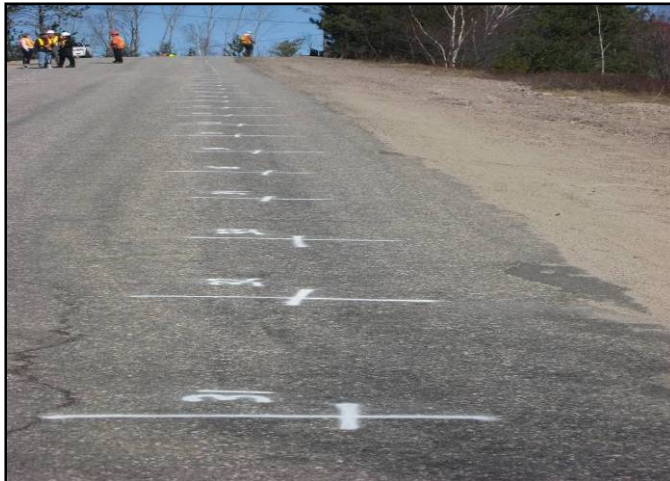
Figure 3.1: Highway 630-Section 1 north bound, 30 test points
