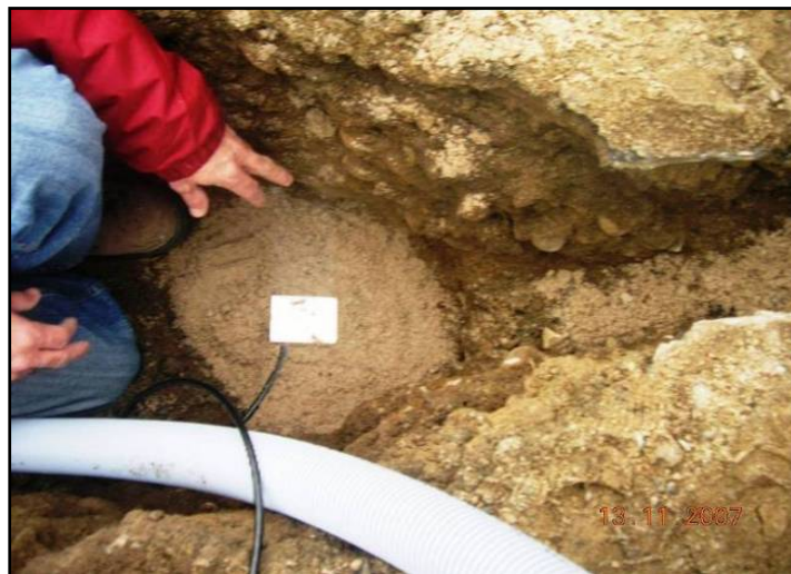
Figure 4.6: The CS-616 probe is inserted horizontally at the subgrade level, Hwy 601
