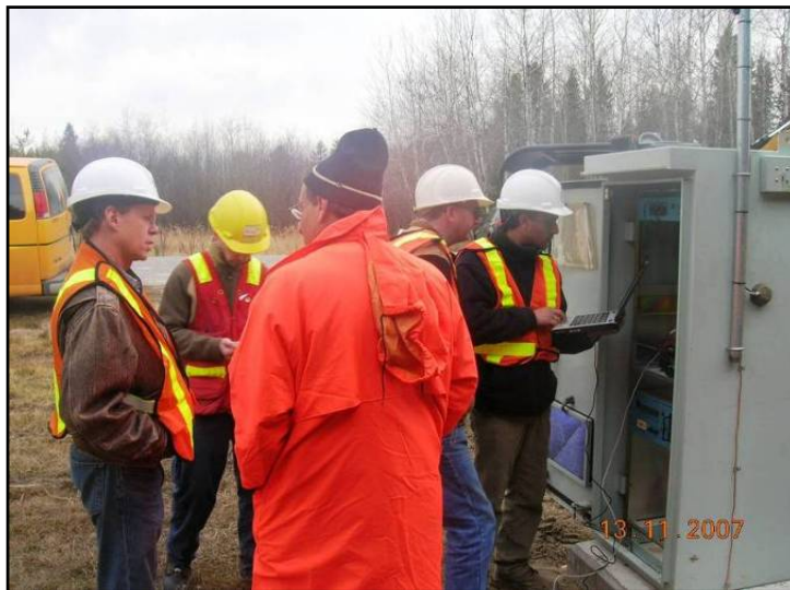
Figure 4.11: Sensors installed, connected to data logger and check-run in progress, Hwy 601
