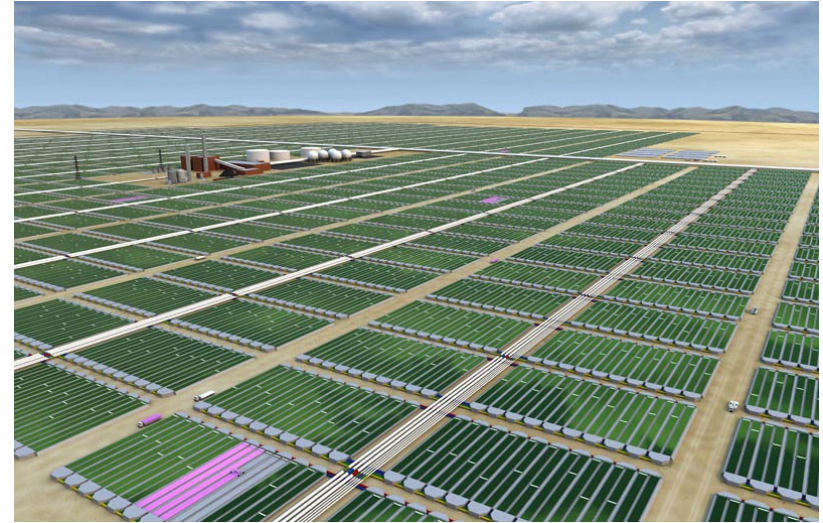
4.26 | Algae Fuel Field A conceptual rendering of a field containing the Solix Algae Photo Bioreactor system, which may be used to produce biodiesel fuel, extracted from the algae grown in translucent tubes.
