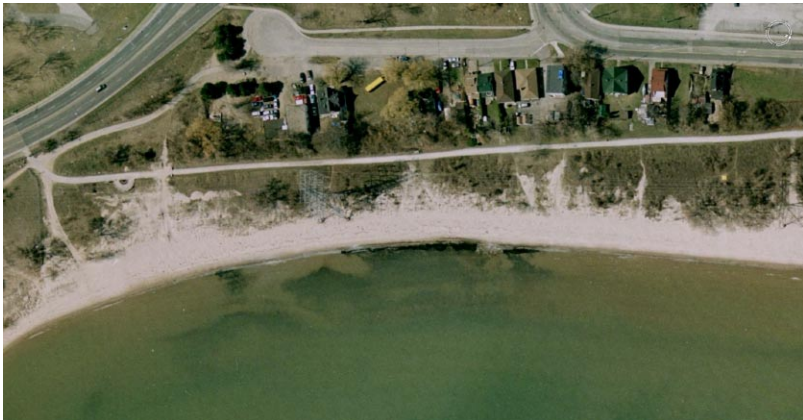
1.22 | Lake Side Powerlines, Aerial
