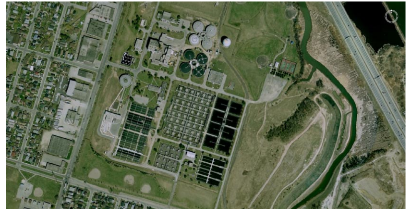
1.24 | Woodward Avenue Wastewater Treatment Plant, Aerial
