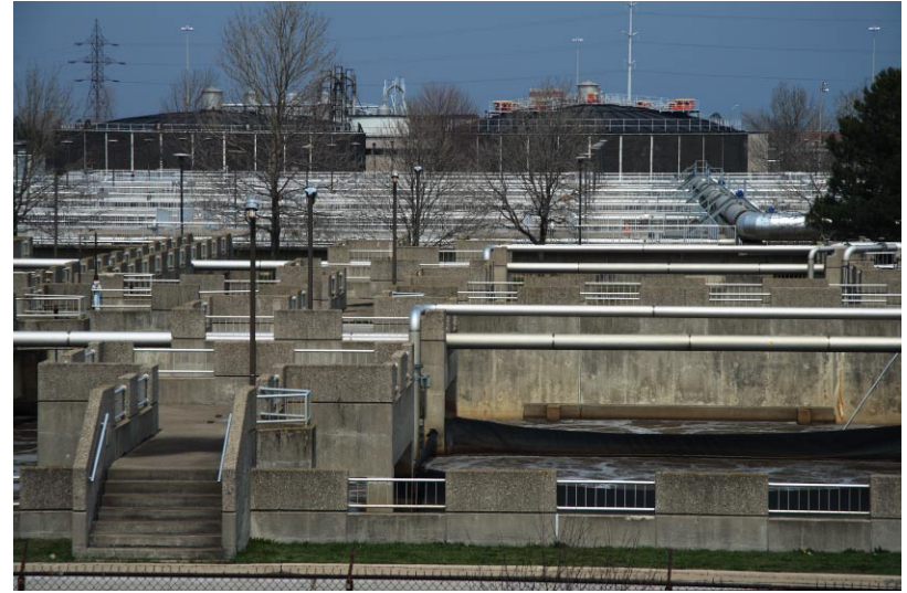
1.23 | Woodward Avenue Wastewater Treatment Plant
