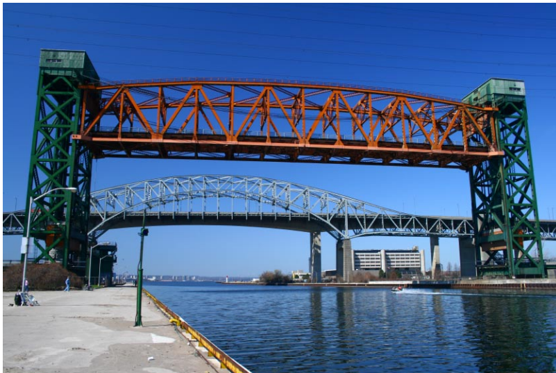
1.39 | Burlington Canal Lift Bridge
