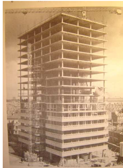
Figure 1.2 Reinforced concrete flat slab building (Cope and Clark, 1984, courtesy of British Lift Slab Ltd.)
