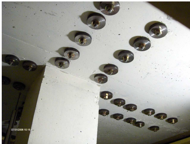
Figure 1.11 bottom view of the slab with shear bolts
