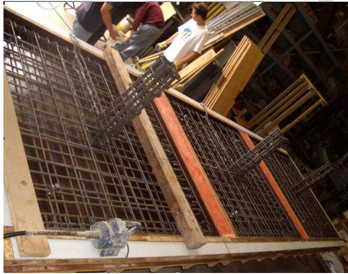
Figure 3.25 Rebar cages and formworks before casting of the specimens
