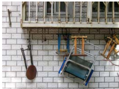
FIG. 4.4 Windows on the first three floors are typically secured with metal frames to prevent break-ins. Residents make use of security window frames to hang their stools and foldable chairs.
