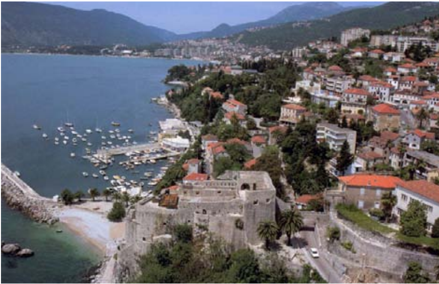
Forte Mare in the Herceg Novi context Fig. 4.78 South fortification of the town in the foreground with cinema and night club established at its roof tops
