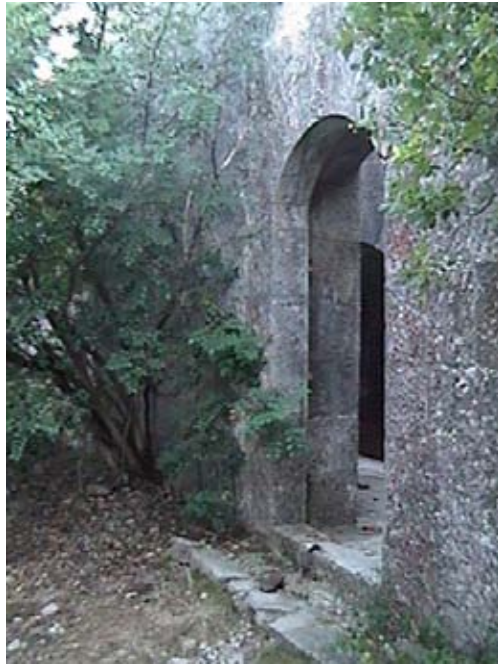
Fig. 4.46 "Gate" to the main complex of Fort Oskoruša
