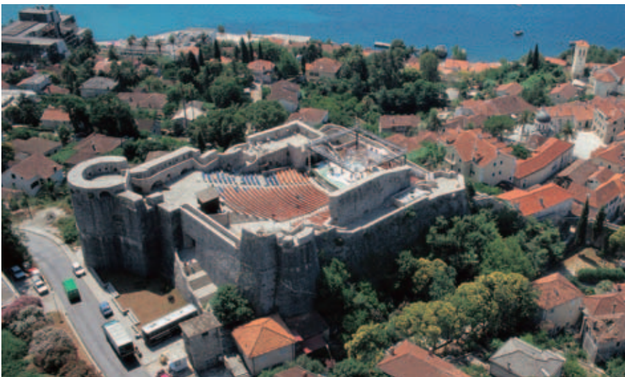
Kanli Fort in the Herceg Novi context Fig. 4.79 North fortification of the town in the foreground with the auditorium and stage at its roof terrace
