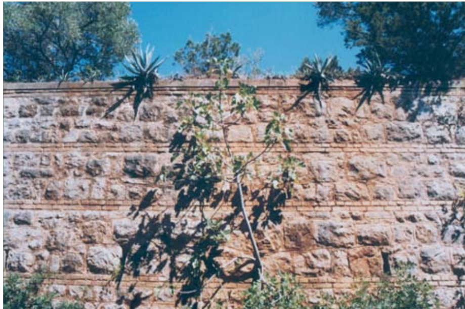
Fig. 4.30 Fort Luštica the trench wall detail
