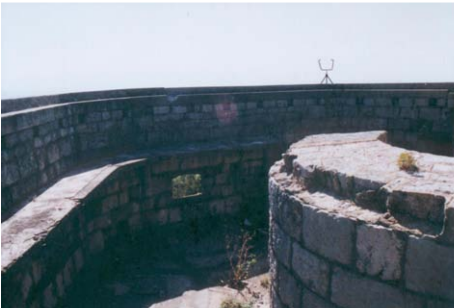
Fort Klinci Fig. 4.28 View of the south-facing hexagon terrace
