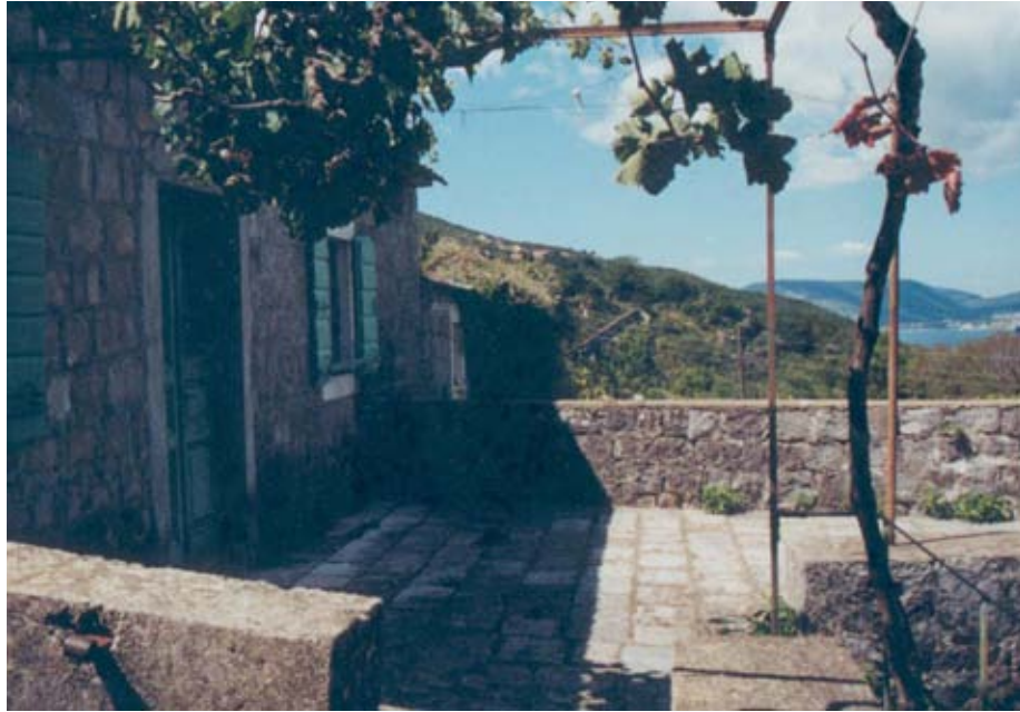
Historical Conditions Fig. 2.100 View of the back stone terrace with wine trellis of an old house in Zabrdje
