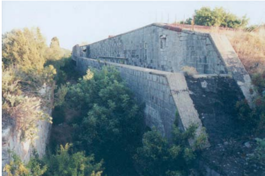
Fig. 4.18 View of Fort Oskoruša looking southeast
