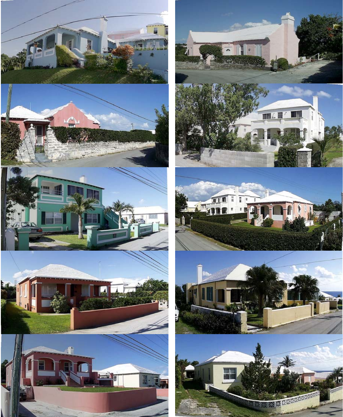
FIGURE 7.5 PHOTOGRAPHIC SURVEY OF SOUTHCOURT AVENUE PROPERTIES
