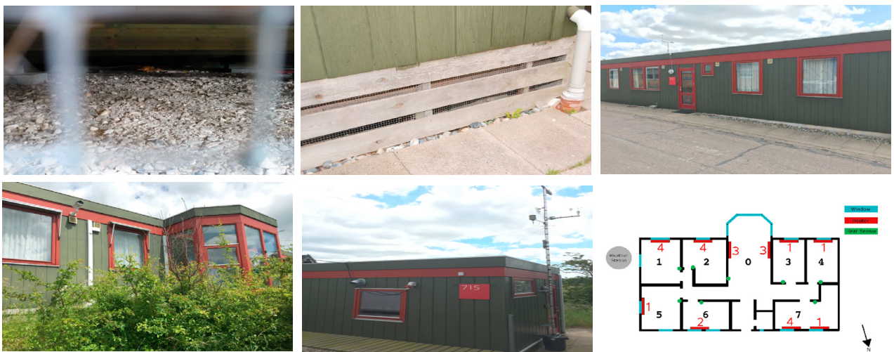
Fig.1. Snapshots of the Flexhouse1: (top-left) Air gap; (top-middle) Planks covering the air gap; (top-right) South façade; (bottom-left) North façade; (bottom-middle) Climate station; (bottom-right) Interior dimensions of the floor plan and sensor distribution
