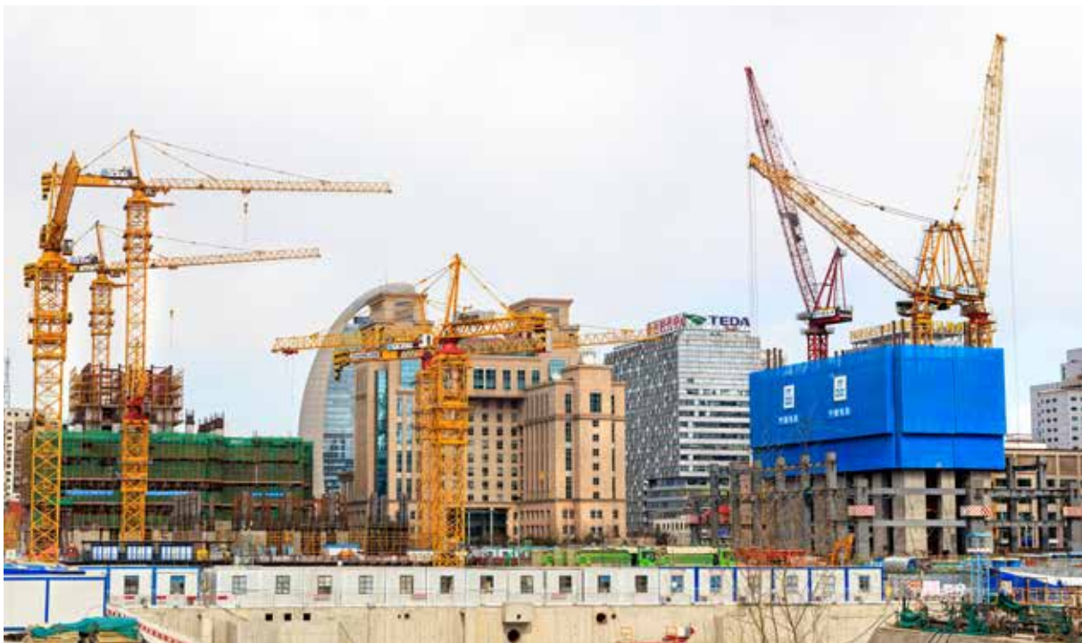
On-going construction are seen around Beijing Central Business District (CBD). testing/Shutterstock.com
