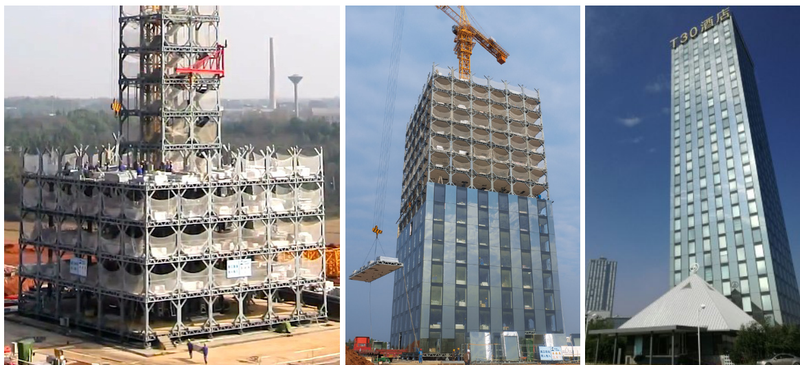
Building Prefabrication Practice of T30 Hotel in Xiangyin of Hunan Province
