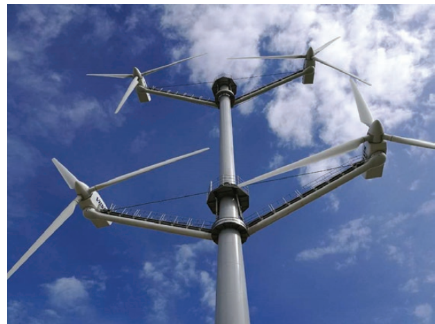
Fig. 2 Multi-rotor wind turbine at DTU Risø campus, Denmark
