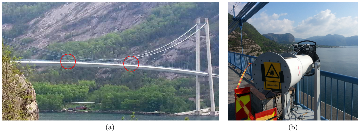
Figure 2. Panel (a): the Lysefjord Bridge is a suspension bridge which was equipped with two short-range WindScanners (two red circles) in May 2014. Panel (b): one of two short-range WindScanners installed on the Lysefjord Bridge providing synchronized scanning of the inflow and wake wind field in a two-dimensional plane at the 55 m bridge deck height.
