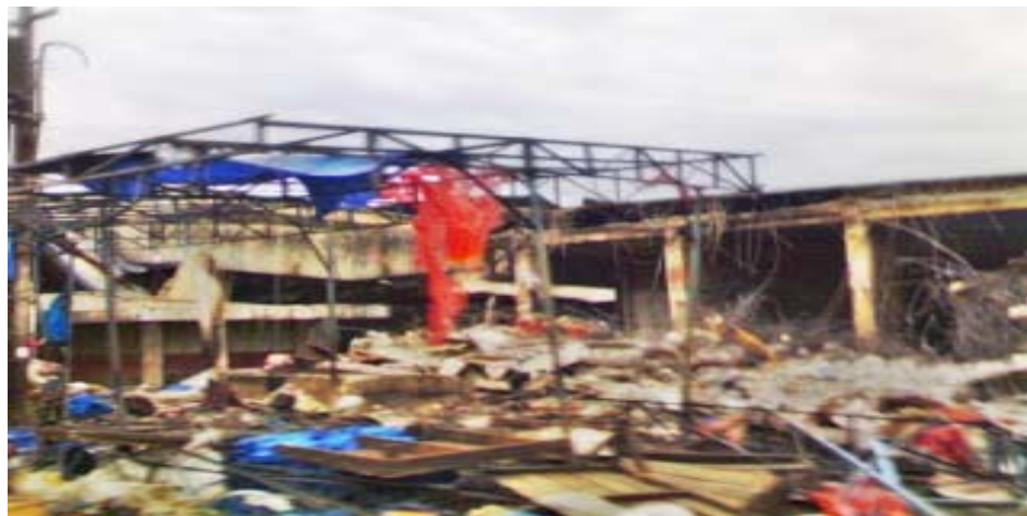
Picture 2. The situation of Pasar Raya Padang after earthquake
