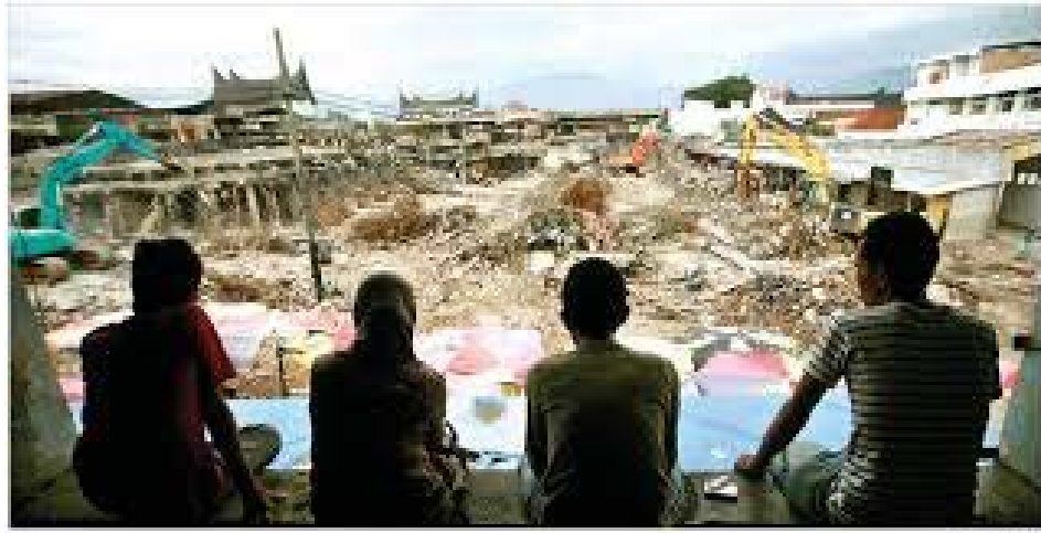
Picture 1. The situation of Pasar Raya Padang after earthquake
