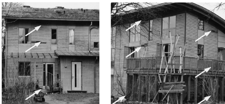
Figure 1 East and South-West orientation of the house facade in Kiel; Arrows point to the location of TMT boards with glued-in electrodes for long-term moisture recording
