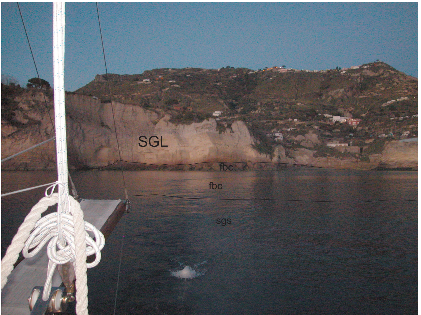
Fig. 5 - The Succhivo tuff coastal cliff. A sketch geological interpretation of the corresponding units is reported based on the geological map of Ischia Island (SBRANA et alii , 2011). The outcropping sequence is represented by the Sant'Angelo Tuffs (SGL). The sea cliff deposits (fbc) have also been reported in their emerged part and they are supposed to continue below the sea bottom, grading to the submerged beach deposits (sgs).
