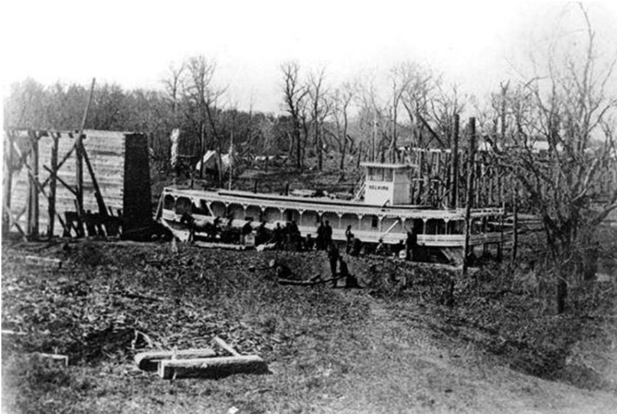
1871-72 – The Selkirk squeezes past the site where the railroad bridge is being constructed across the Red River. Behind the boat, frame buildings are going up in the newly born Fargo.
