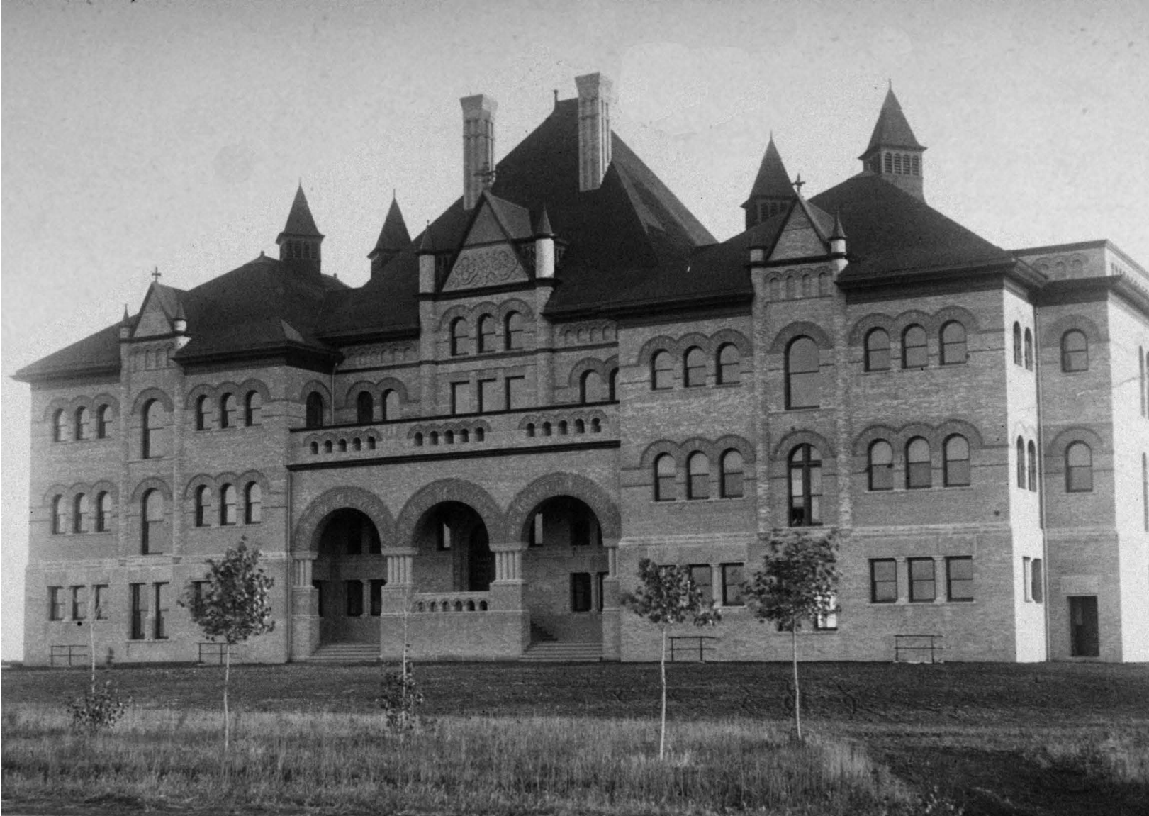
The Normal School's original building in 1888.
