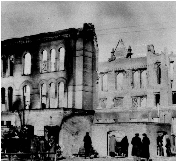
Salvage work begins on the power plant, while classes are held in Weld, the dormitories, and nearby homes.
