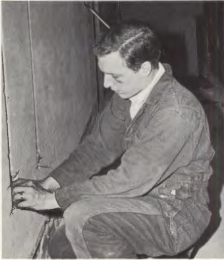
Doing our own wiring saves the school money.
