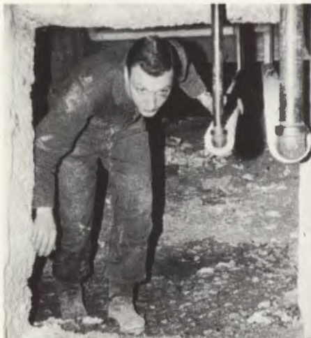
Much of the wiring requires underground work.
