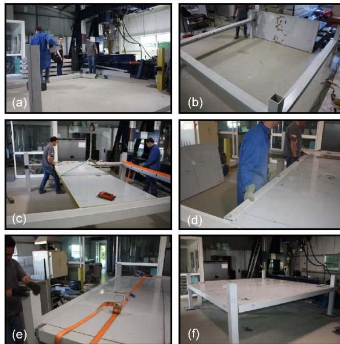
Fig. 8.17. Stages of the assembling process: (a) placing columns; (b) connecting beams to the columns; (c) mounting panels along beam-panel connection; (d) placing panel-panel connector; (e) installing the last beam; (f) final prototype.
