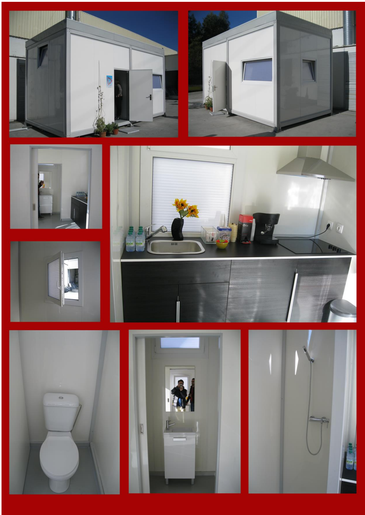
Fig. 3.2. Temporary single-story prototype.
