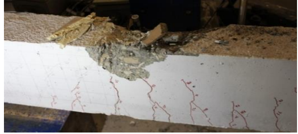
b) Crack pattern at failure load of the R-7S-R beam
