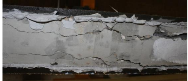
d) Crack pattern in the bottom surface at failure load of R-3L beam
