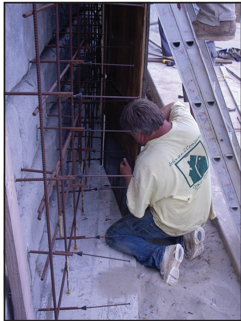
Grant Goldberg fits the rebar through the wooden panels, creating the form for pouring the concrete walls.
