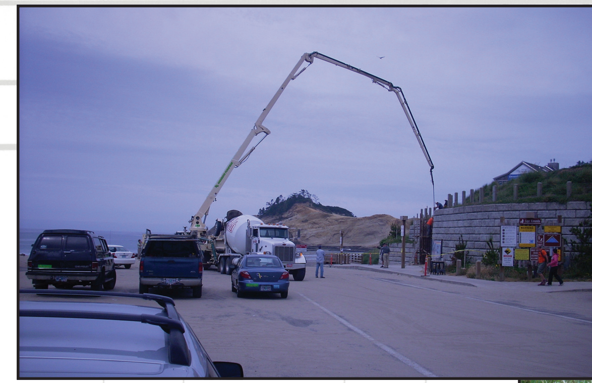
Concrete is pumped into the form.
