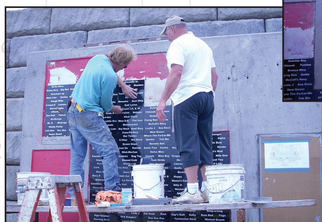
Dan Eddy and Albert Knopf attach tiles to the concrete wall.
