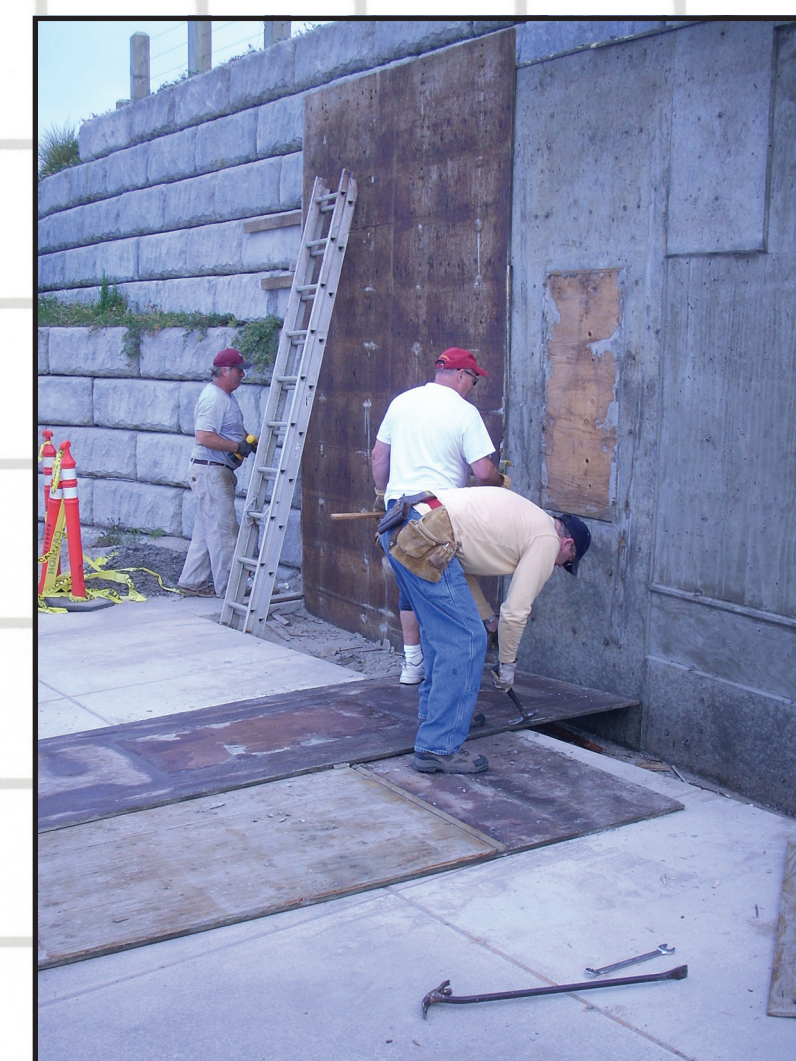
Darrin Richard (L), Albert Knopf (C), and Jeff Raines (R) pull the form away after the concrete has set.
