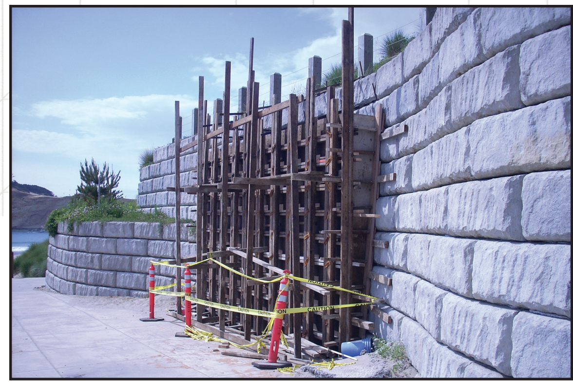
The form is in place and ready for concrete.
