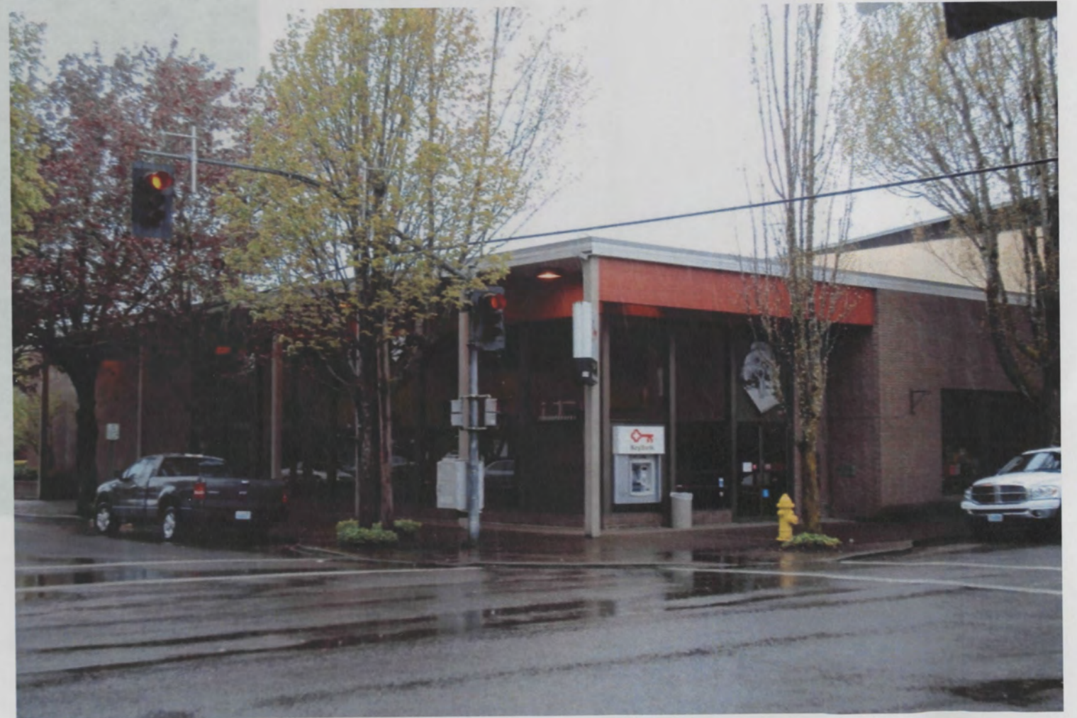
Above: Key Bank, 2012 Photo Credit: Jordan Mixsell
