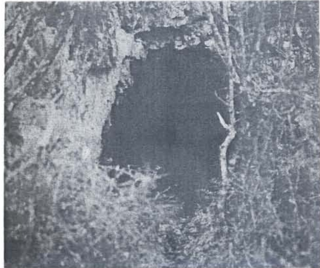
Fig. 6. Present state of the adit D-3
