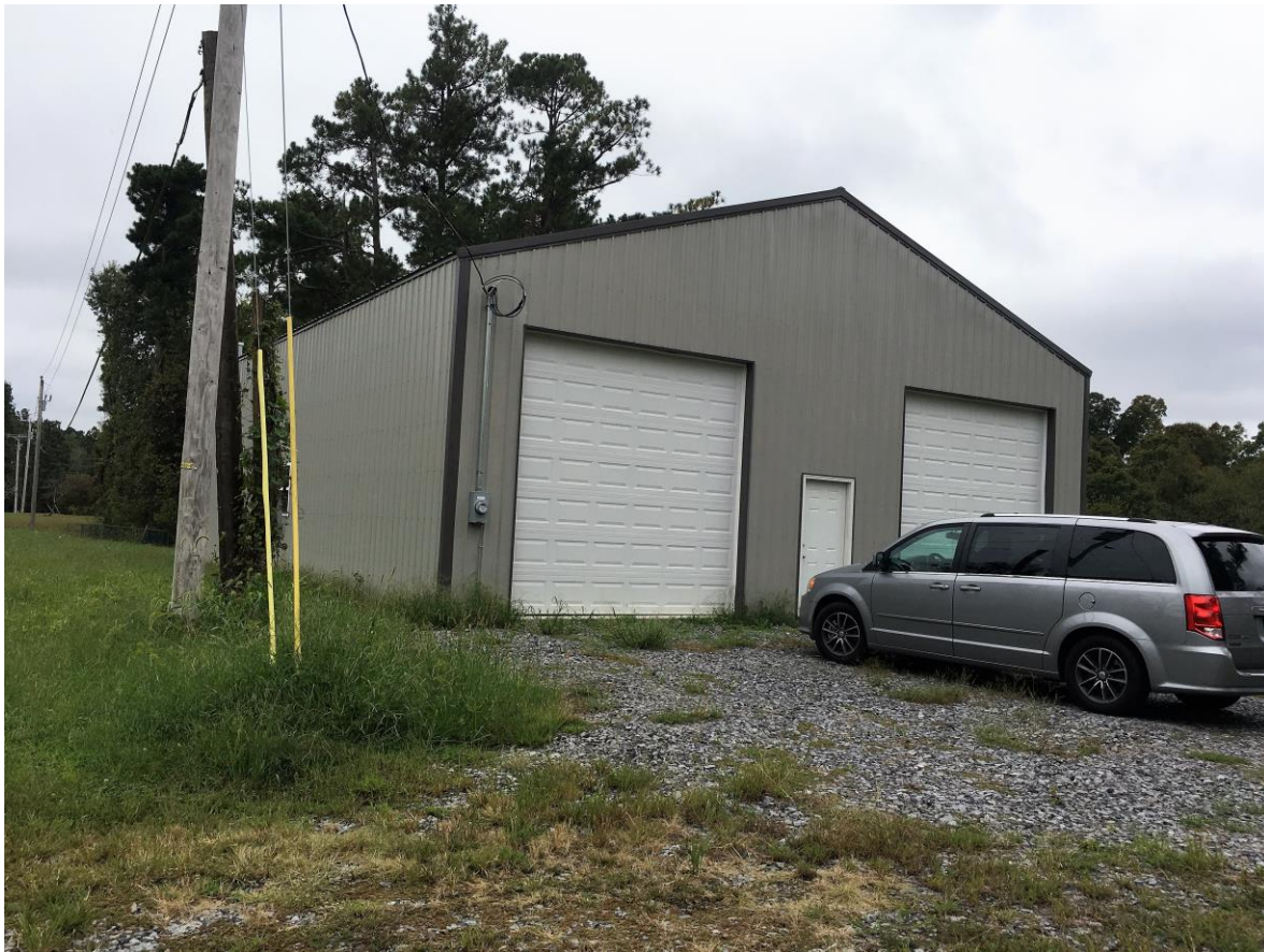
Figure 13. The large shop building contains an oven and stove, two deep large freezers for pelts or meat, two industrial sized refrigerators, and one full bathroom.
