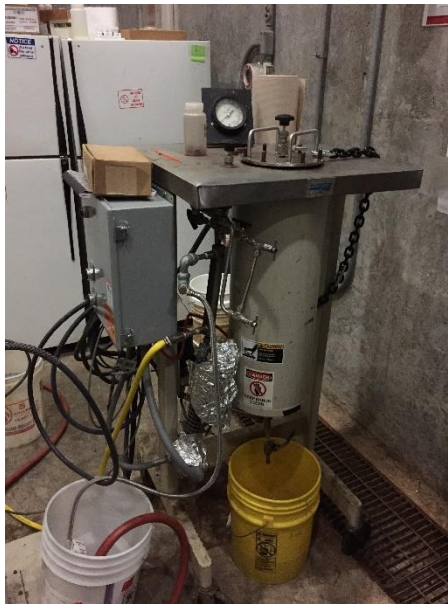
FIGURE 3.1 – Percolating reactor used for hydrolysis
