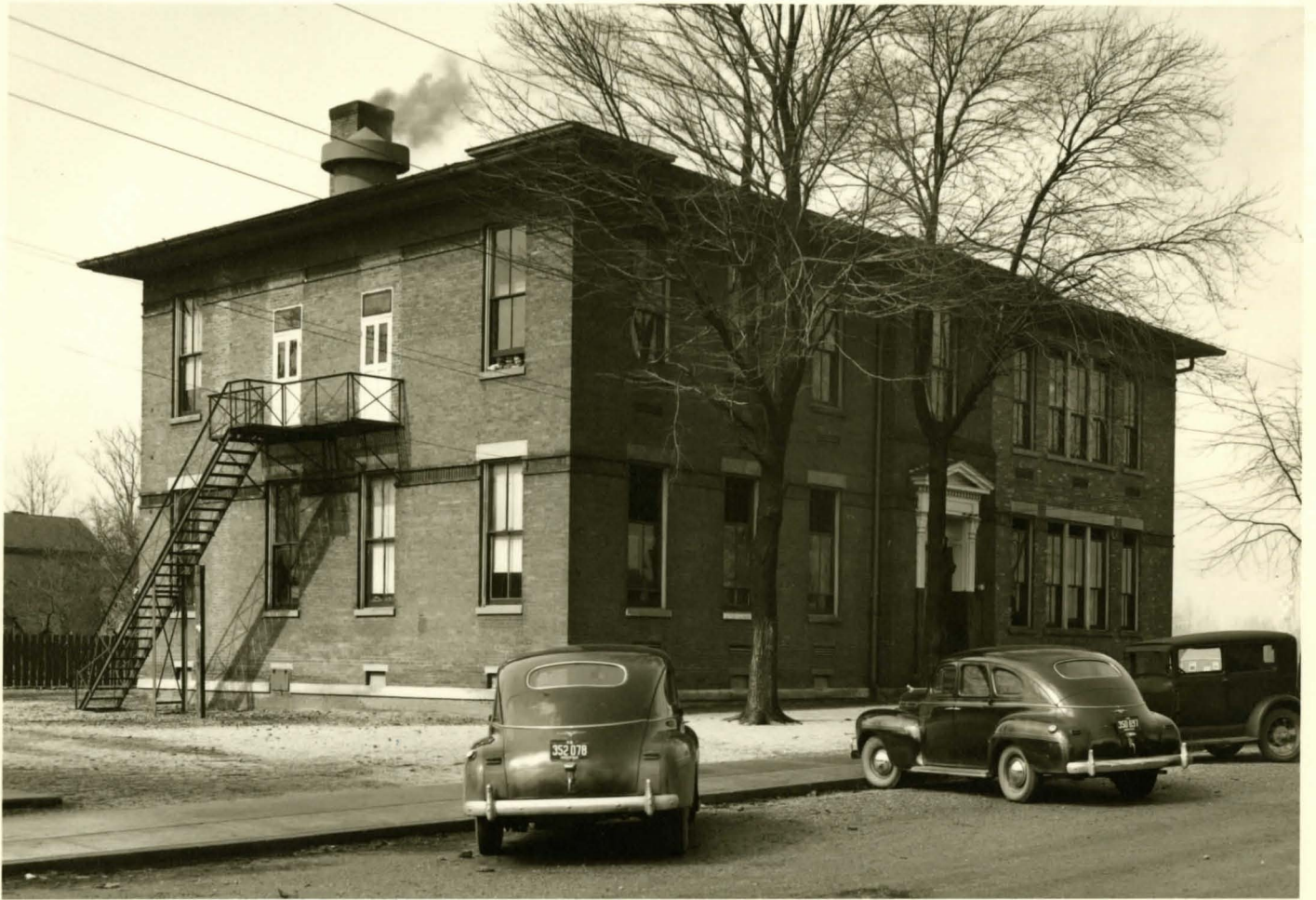
Port Fulton School Building built 1880
