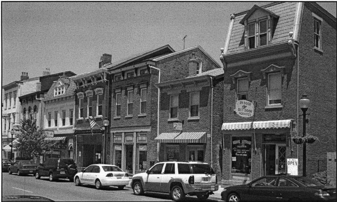
Figure D.5. Business and Streetscapes along Monmouth Street.
