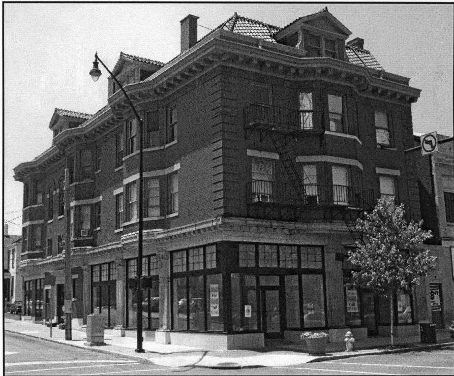
Figure D.6. Marx-Cromer Building at Ninth and Monmouth Street.
