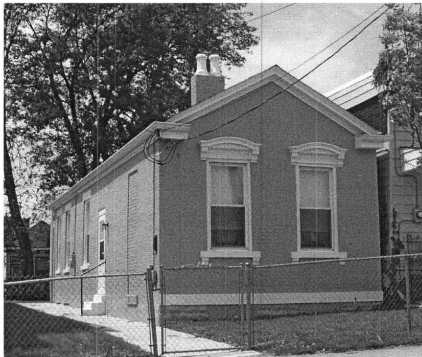
Figure 4.27. 1136 Central Avenue Rehabilitation.
