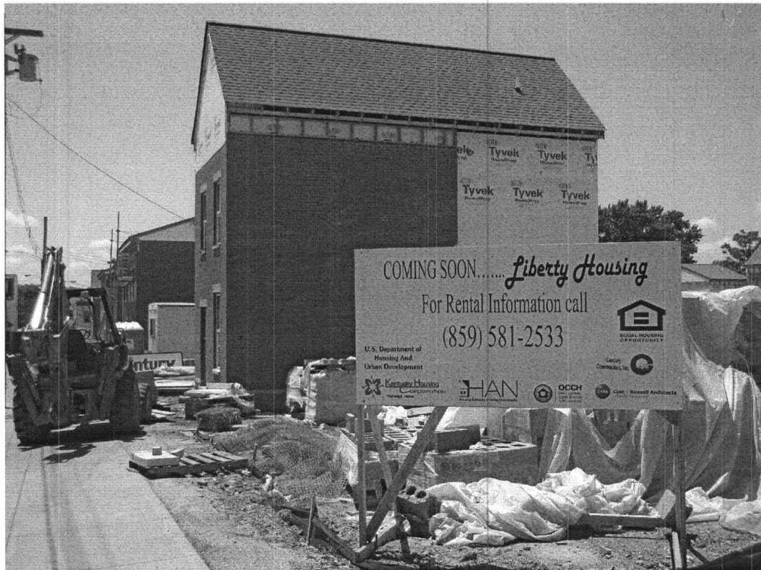
Figure 4.20. Additional photo of Liberty Housing, Phase II, under construction.
