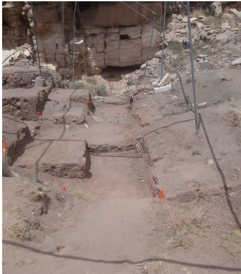
Figure 4. GR-2 viewed from the site's south end. Source: author photo.
