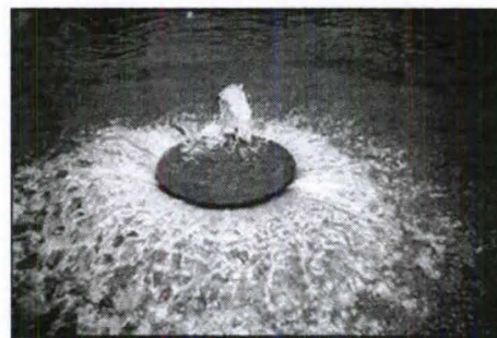
Figure 1.3 - Sanitary Sewer Overflow (Source: EPA)
