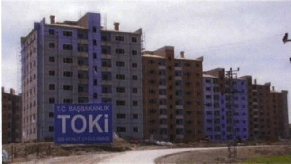
Figure 6 TOKI construction zone
