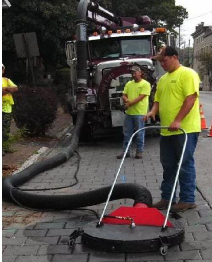
Figure 14. Hydro excavator method (a) Prototype attachment (b) Hydro excavator truck
