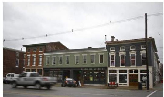
Figure 5. The former Wayside Christian Mission block on E. Market St
