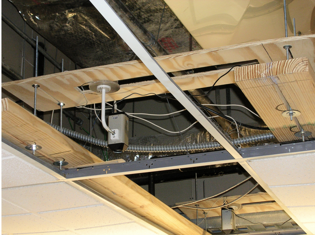
FIGURE 12–Mounting platforms that hold cameras. Slotted regions allow the cameras to slide anywhere along the platform.
