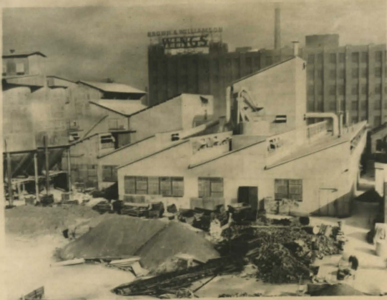
Fig. 4. General plant view showing part of ventilating system with collectors
