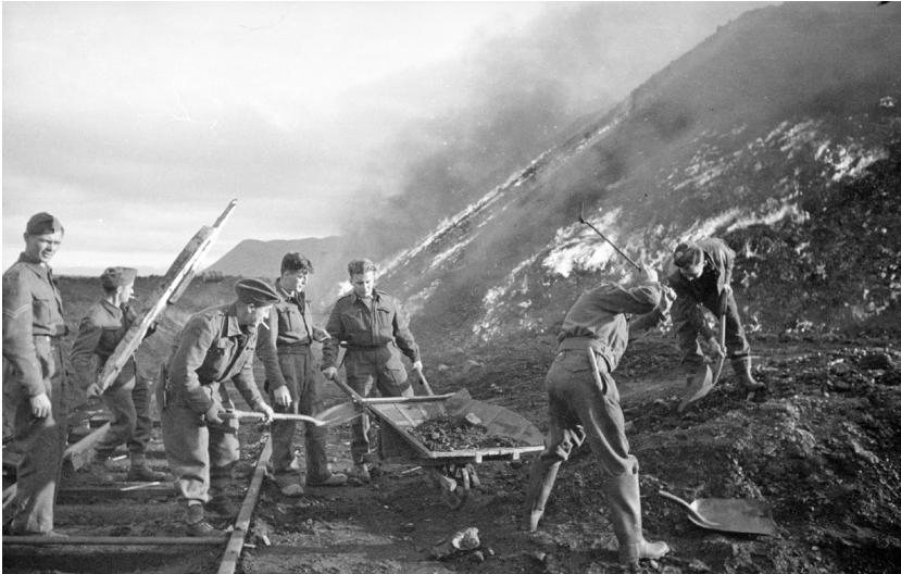
Royal Canadian Engineer sappers fire the coal pile at Barentsburg. [Library and Archives Canada PA-180524]
