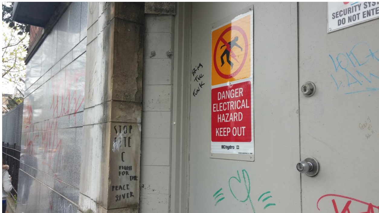
Fire hazards (photo: C. Sandilands)
